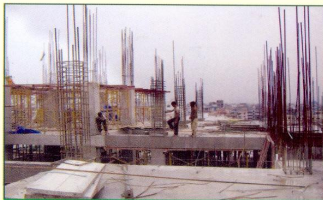
Under construction 14 storied 182 flats at Lalmatia, Dhaka
