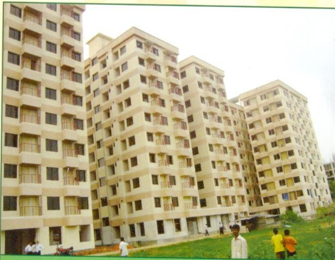
Newly Constructed 10 storied 108 flats at Haliashahar, Chittagong
